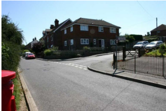
Picture 2: In Barden Road, junction with Northfields
