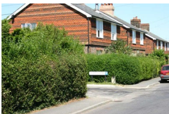
Picture 9: In Northfields, junction with St Mary's Lane
